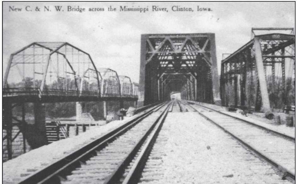
1909 - New double-track C&NW is completed. Single track on right was in service from 1865-1909. Left: Clinton-Illinois Wagon Bridge 1891-1954
