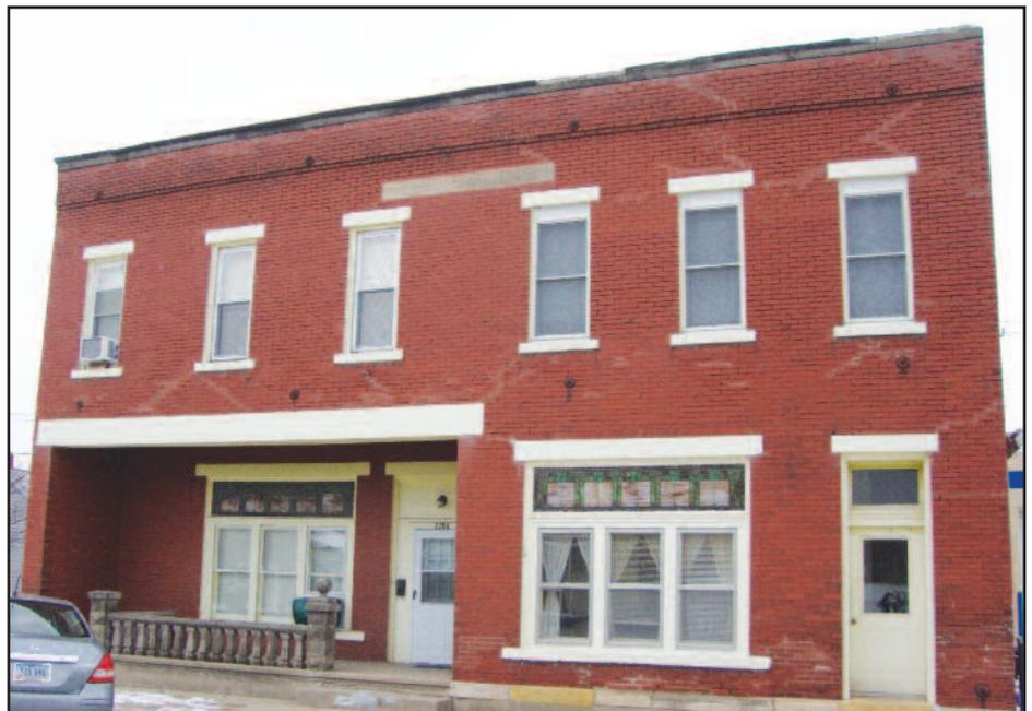
**THE BRUINS** was built in 1913 and its exterior has the same appearance today in 2013. The vintage photo above taken of the Leslie family in August 1913 was on the front porch. The concrete balustrade is still intact. The plate-glass windows installed in 1913 have been replaced with sets of three individual ones and topped with stained-glass transom windows. Currently, the 4-unit apartment building is owned by Linda and Robert North.
