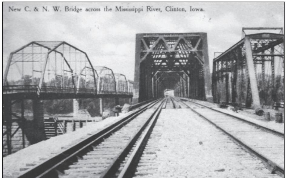
1909 - New double-track C&NW is completed. Single track on right was in service from 1865-1909. Left: Clinton-Illinois Wagon Bridge 1891-1954
